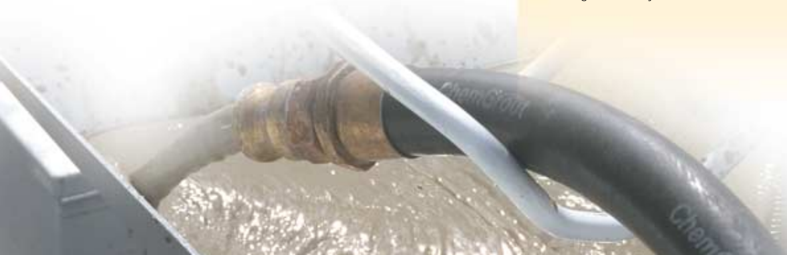
BentogROUT being injected to seal a below-ground utility manhole.
