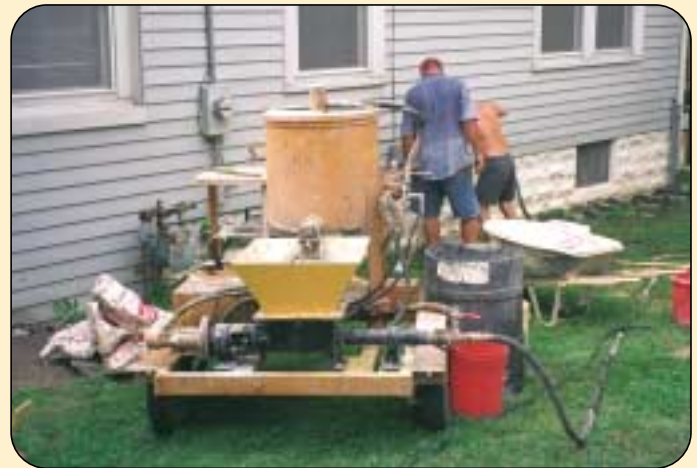
Chemgrout CG-555 trailer mounted pump with mixer.
